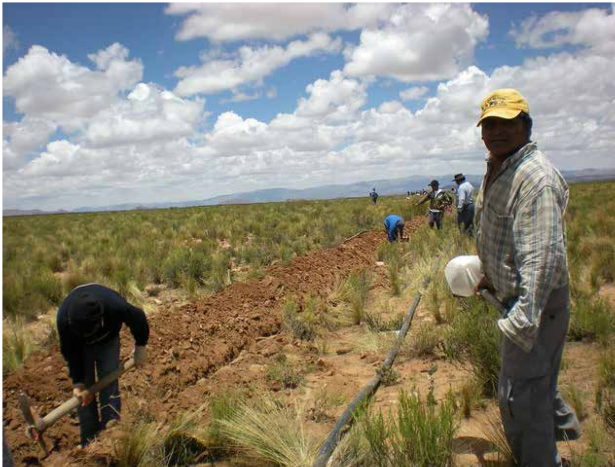
Long months of community work to install pipes to bring water from rock glaciers to indigenous villages in the Puna region in northwest Argentina served to strengthen collective organisation and community ties in an inhospitable ecoregion, where solidarity and joint efforts are essential to daily survival. Credit: Courtesy of Julio Sardina
