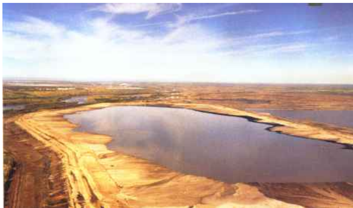
Alberta Tar Sand, constructed toxic effluent pond
