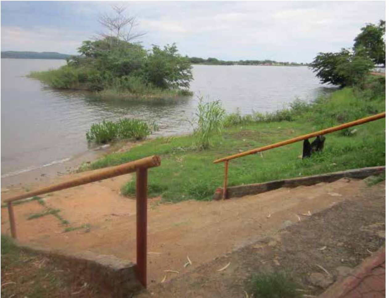
Access stairway to the Tocantins River in the central Brazilian state of Tocantins, which no longer has flowing water since it was dammed to generate electricity, mostly to be used in other parts of the country, and which contributes very little to local development. Credit: Mario Osava / IPS
