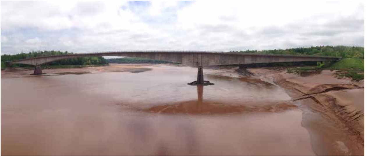
The Gosse Bridge, that stretches over the Shubenacadie River and the remnants of the old railroad bridge.
