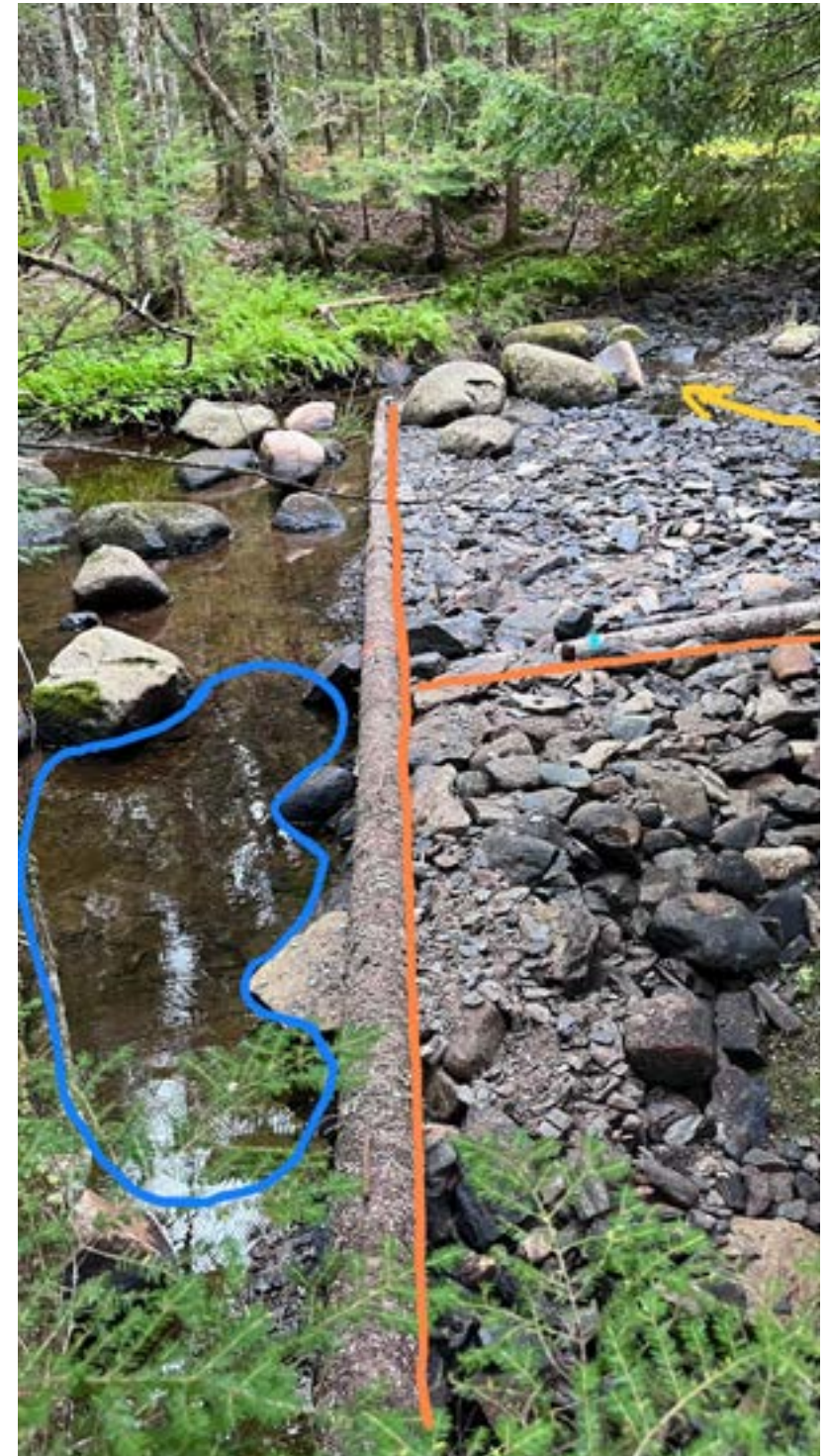
Figure 2. Example of a digger and deflector log (orange) installed in a stream using the flow of water (yellow) to dig out the pool below (blue). Image Credit: Veres, J. 2022
