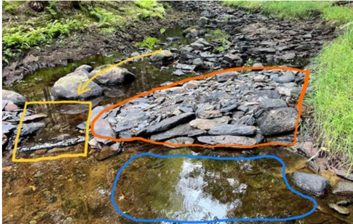
Figure 3 Example of a newly constructed rock sill (yellow box) with the pool (blue) just below the rock wall (orange). Image Credit: Veres, J. 2022
